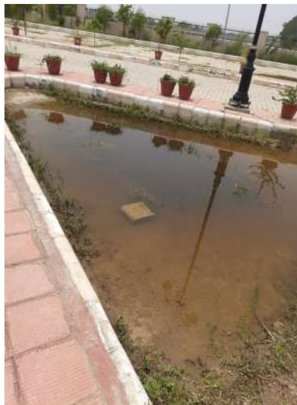
Fig. 2.5 Rain water harvesting system II located near car parking area
